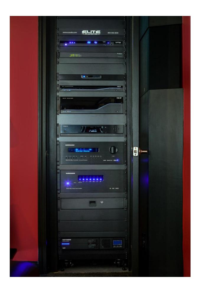
The equipment rack is set into the back corner of the cinema, housing the AudioControl gear, power conditioning and more — all actively cooled for reliability and longevity.
